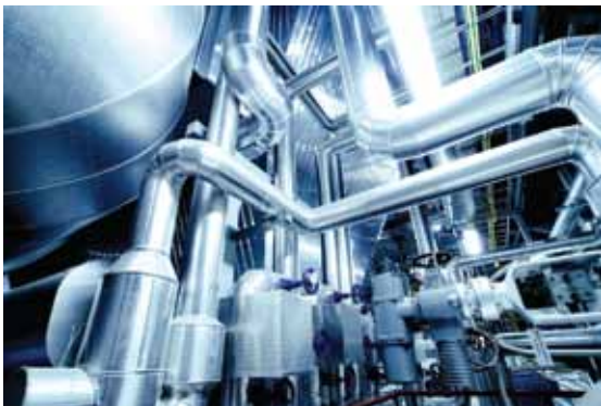
Non-contact density measurements through the installation pipe
